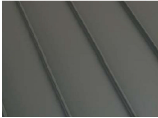
STANDING SEAM METAL ROOF TOWER GABLE WESTERN "CHARCOAL GRAY"
